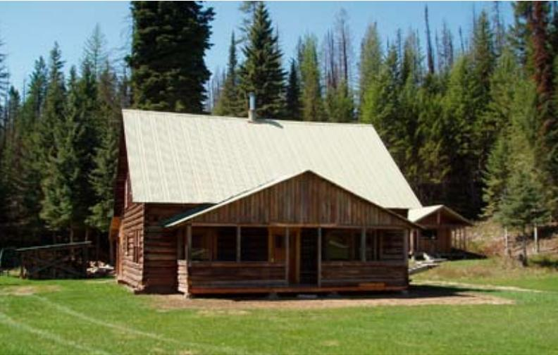
Figure 10—Standing-seam roof.
