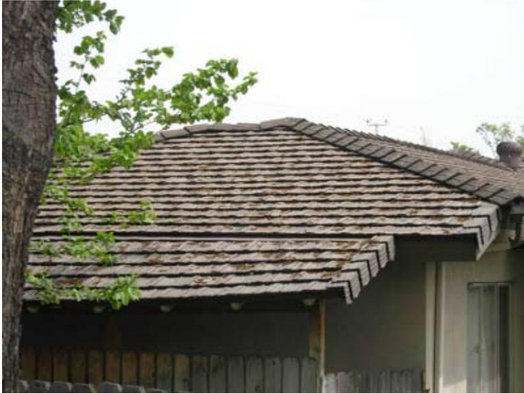
Figure 14—Concrete tile roof.
